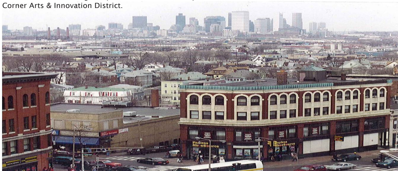
The Pierce Building shown with Downtown Boston in the distance.
